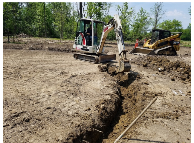
Pictured: Staff working on drainage improvements at Gerspacher Park
